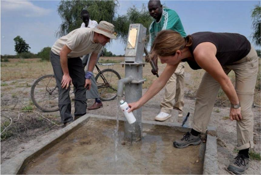
**Fig. 2.** Handpump water well for the local rural water supply, Type *Ajay*, *India-Mark II*.
