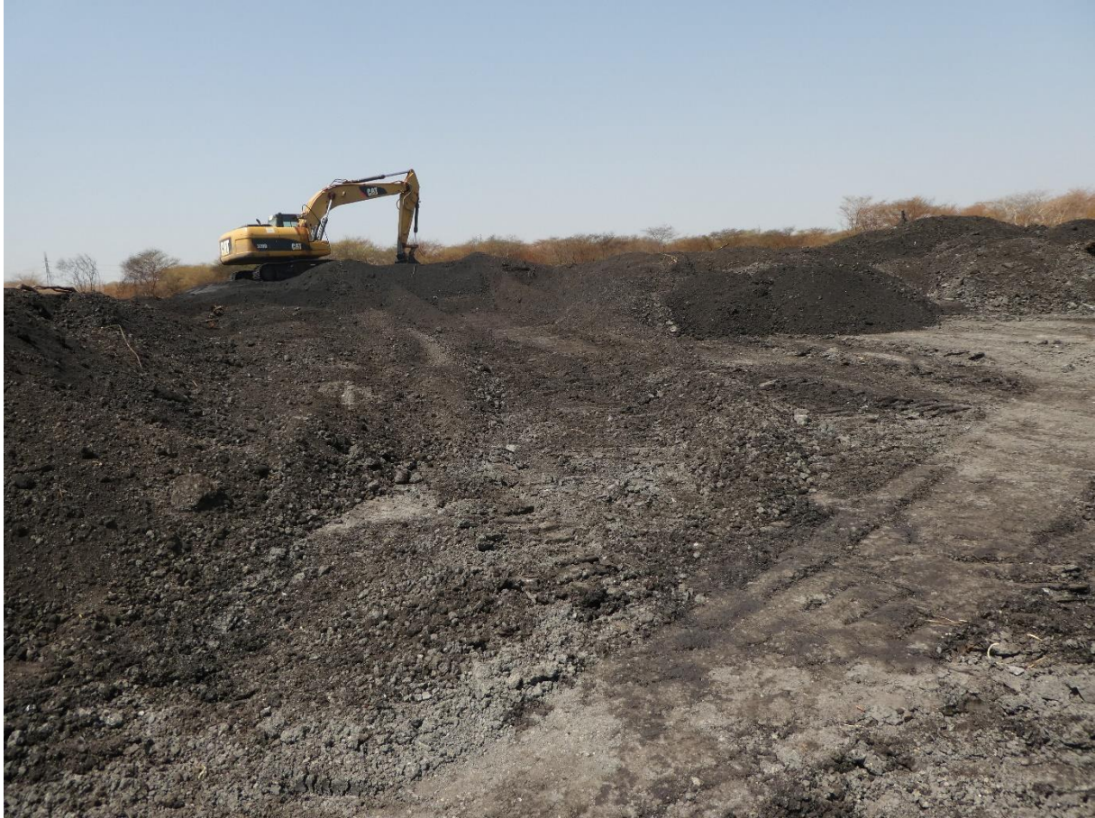
Figure 28: As of the time of the on-site investigation, heavy equipment was still to be found on the site of oil spill 2. Bulldozers were used to remove a layer of the soil and to shove it into mounds. Noticeable are the various colors of the soil in the mounts. The black piles are presumably comprised of oil-saturated earth.
