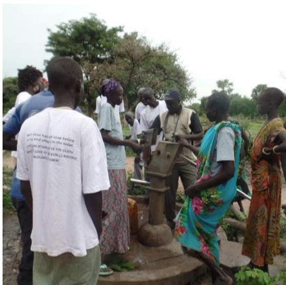
Minor repairing in Citcok Borehole, Cueibet County
